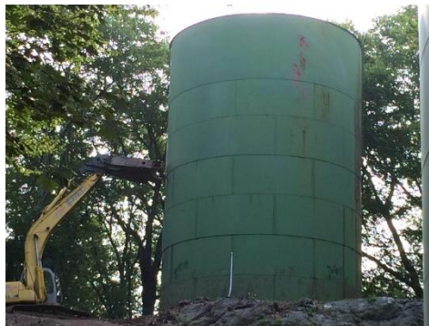
The Grove Street Water Storage Tank was demolished in July 2015.
