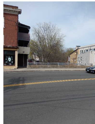
Figure 17: Private properties abutting the Pequabuck River
