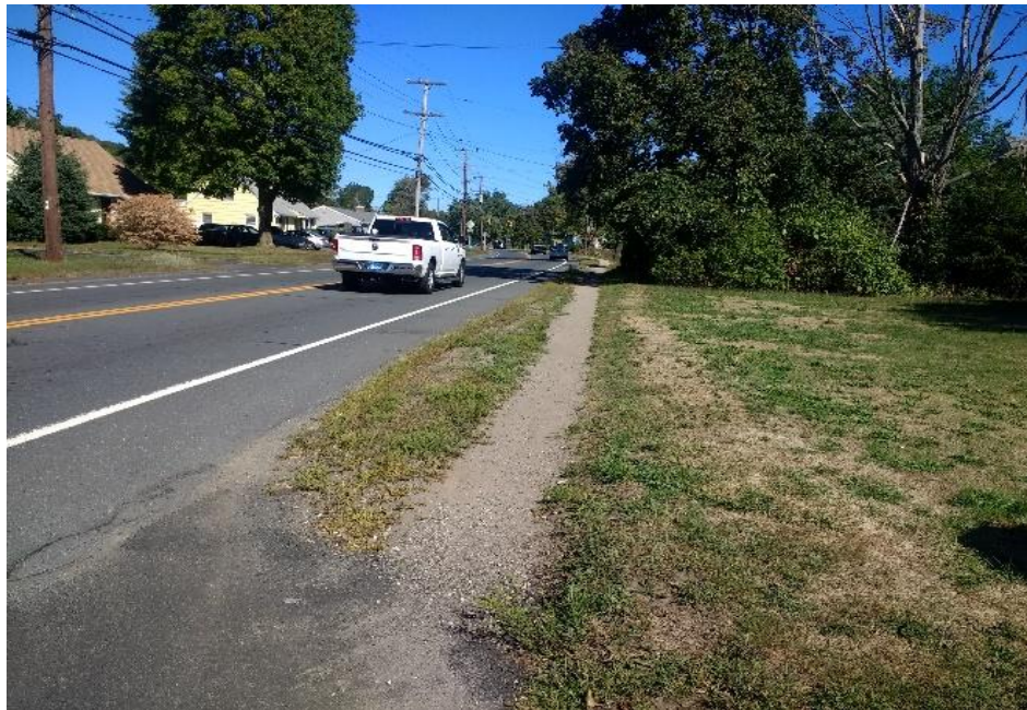
Photo 8 Worn Path example North of New Street
